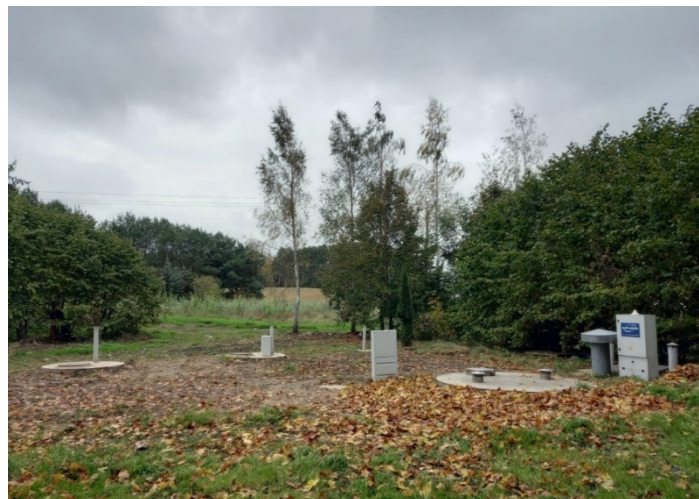
Figure 3: Mechanical-Biological WWTP: Bioekol Mini 75, in the Bure Misie Settlement (photo: Pluciennik M., BMCF)
