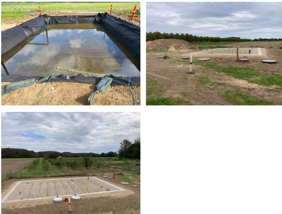
Figure 3: Pictures of the plant during construction (photos: Danmarks Naturfond).
