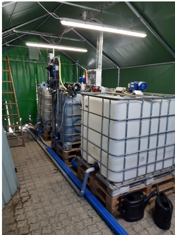
Figure 2: Pilot plant to test nano bubble technology (photo: Morten Lykkegaard Christensen).
