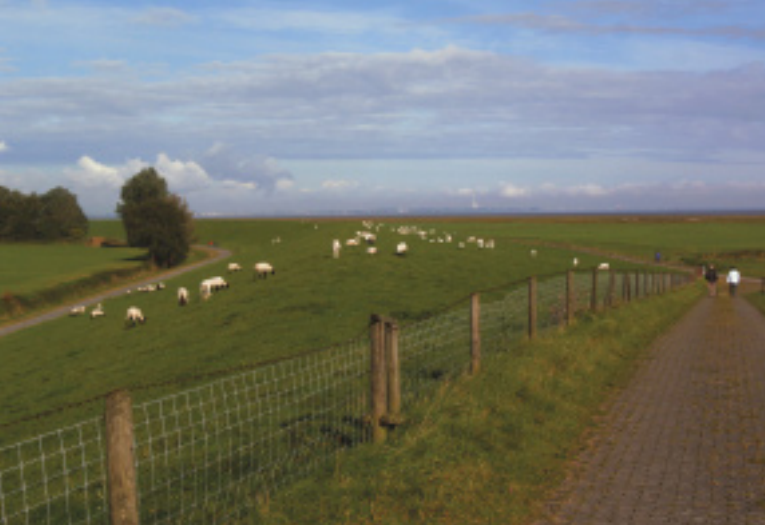
Dyke in Varel, Jadebusen between Wilhelmshaven and Bremenhaven (Photo: Frank Ahlhorn)
