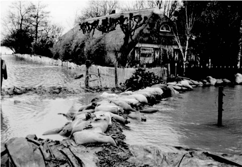
Fig. 1. Dike reinforced with sandbags - January 1995 (photo by Rijkswaterstaat DWW, Delft).
