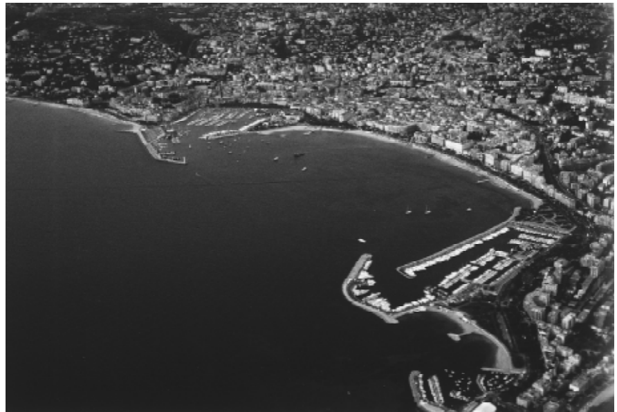
Fig. 2. Yachting harbours and reclamation fill structures on the French Riviera. Vertical photograph shows St. Laurent du Var and the Var river mouth. Much of the airport platform on the right adjacent to the river mouth consists of land reclaimed from the sea through infill of the shallow (< 30 m) submarine slopes of the Var Delta. Oblique photograph depicts yachting harbours on either side of the Cannes urban-front beach, regularly nourished since 1965. Note the small artificial beach on the lower right between two yachting harbours.
