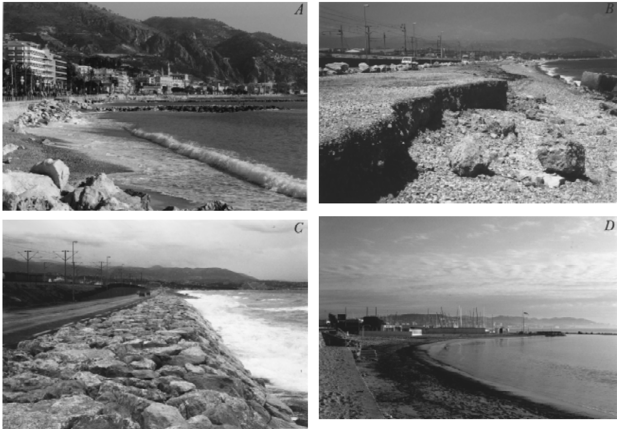
Fig. 3. Photographs of French Riviera beaches, depicting some of their handicaps, such as narrowness, chronic erosion, dominance of gravel in their sedimentological composition, heavy and sometimes inefficient beach stabilization structures such as rock armouring, groynes and seawalls (note the vertical wall in A), and pollution of low-energy sectors by seagrass driven onshore. A. Menton; B. Villeneuve-Loubet; C. Antibes; D. Cannes.
