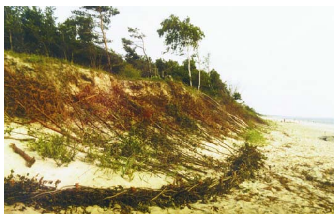
Figure 2: Eroded foredune fastened with fences and fascines in Pajuris regional park. Photo: E. Paplauskis, June 2001
