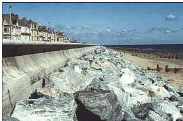
Fig. 8: Promenade of Withernsea, seawall and rip-rap.
