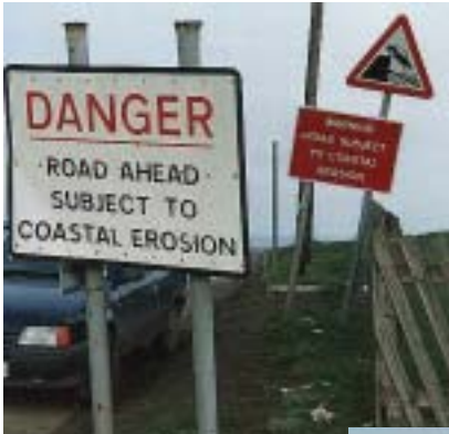
Damage to infrastructure
