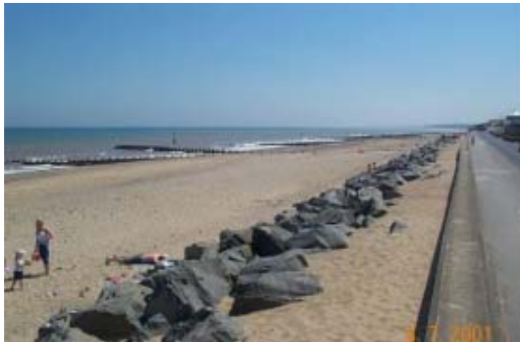
Fig. 02: Wooden groins, seawalls and boulders at Hornsea.
