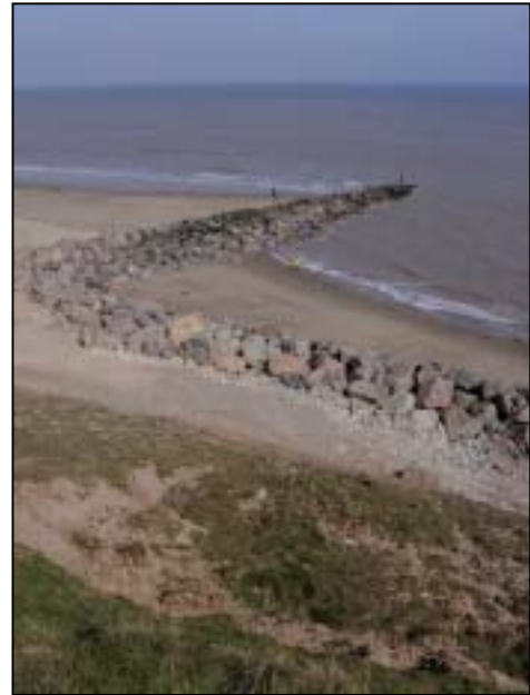
Fig. 03: Rock groin and revetment at Mappleton.
