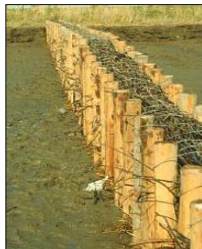
Fig. 10: Pier protection of tidal area.
