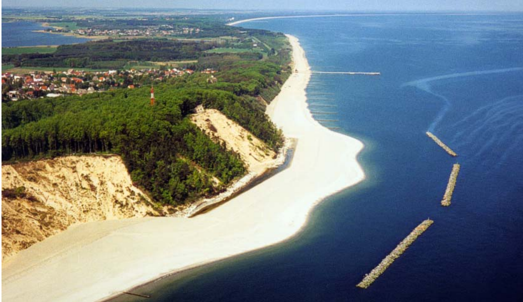
Figure 4: Coastal protection/flood protection works with a system of offshore breakwaters, groins and beach nourishment at the Streckelsberg / Usedom Island (Photo: Dr. B. Gurwell).
