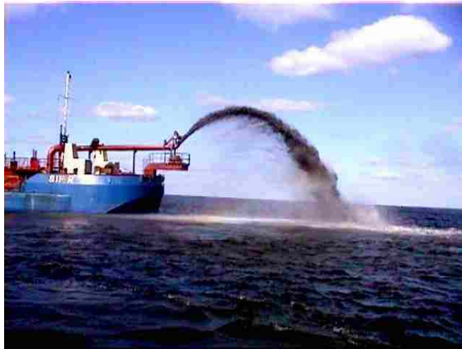
Figure 3: Submerged nearshore nourishment at the Lithuanian mainland coast. Photo: V. Kaunas, April 2001
