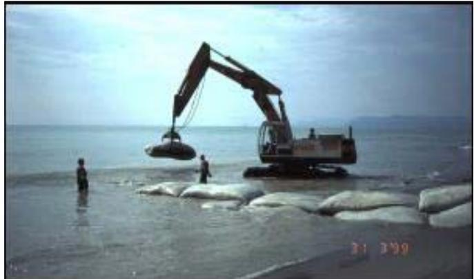
*Figs. 13, 14 & 15: Sand bags and construction works of experimental submerged groins.*
