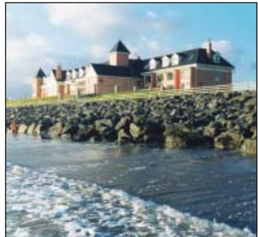
Fig. 6: Armoured section at Sand House Hotel.
