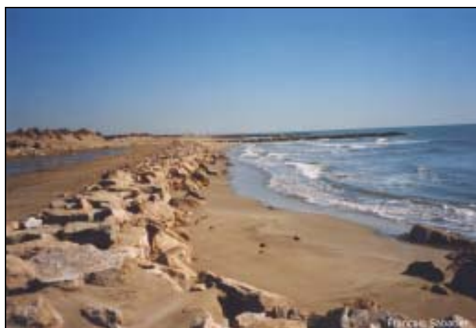
Fig. 22: Seawall and battery of groynes in the Petite Camargue.
