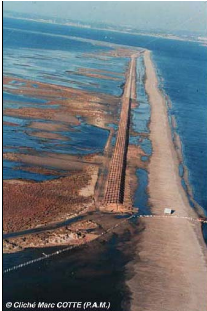
Fig. 17: Rebuilding the dune ridge of the Gracieuse spit.
