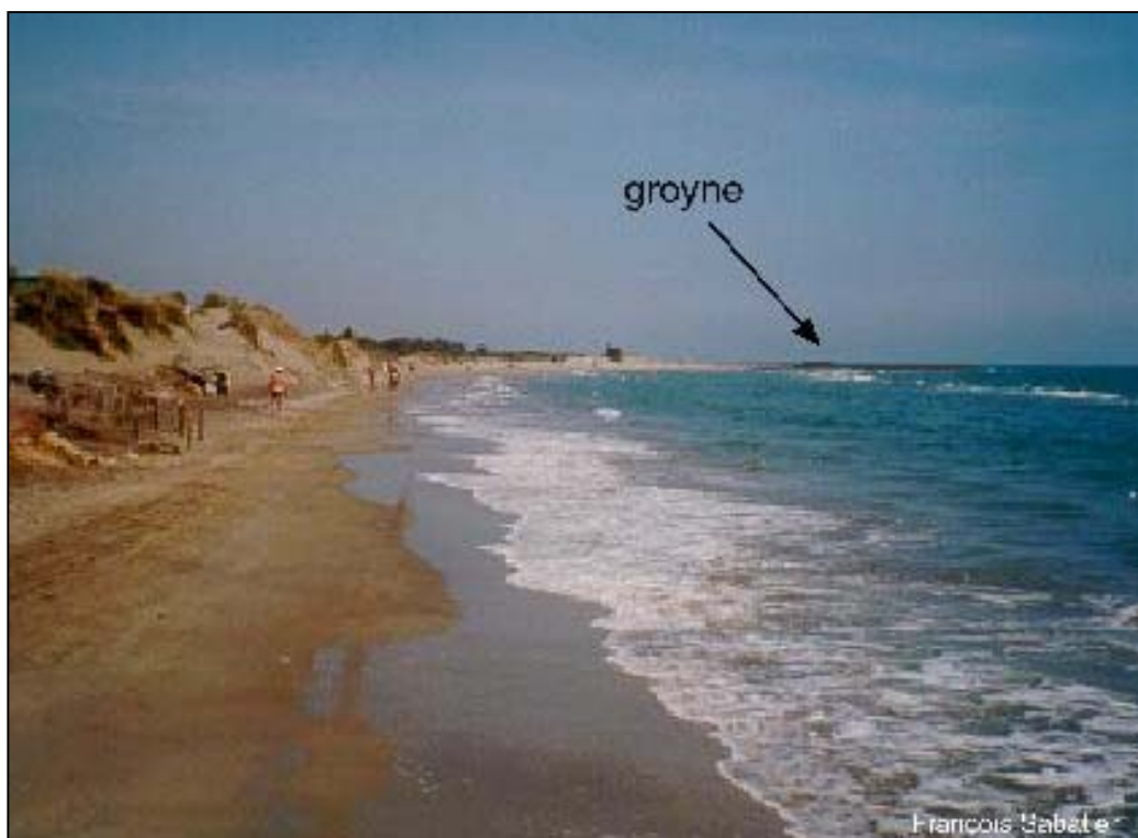
Fig. 29: Erosion downstream from a battery of groynes along the drift direction
