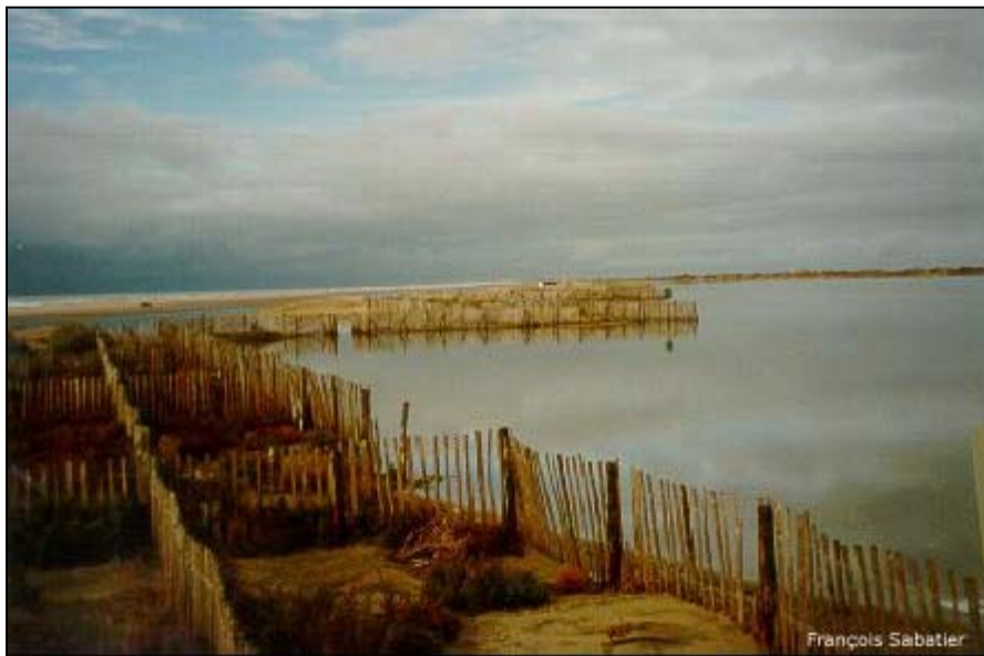
Fig. 25: Temporary lagoon formed by installation of ganivelles in middle of beach.
